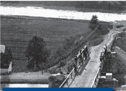
Pontoon Bridge Location
