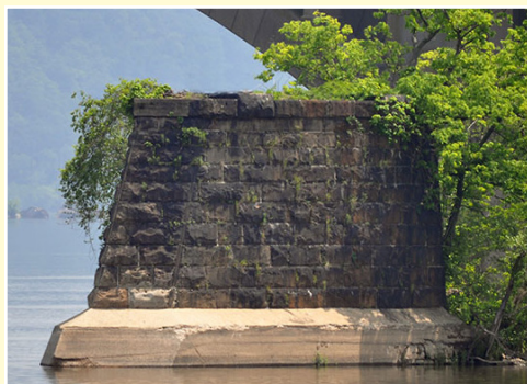
Original Bridge Support
