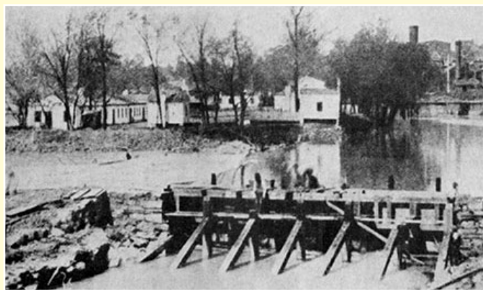
The site of disaster; the small workshop buildings of the Brown's Island laboratory. This photograph was originally identified "The Laboratory For Small Ammunition At Richmond."
