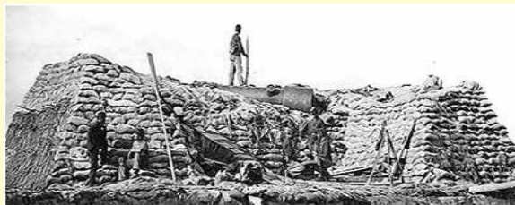
After explosion - This was the appearance of the Marsh Battery after the "Swamp Angel" burst while firing its 36th round at Charleston. The breech was blown off and the gun pitched forward. (Illustration from "Battles and Leaders.")
