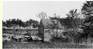
Ellerson's Mill on Beaver Dam Creek (LOC)
