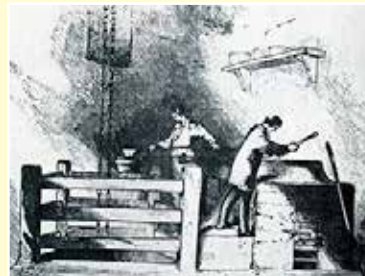
Workers shown in this 1853 engraving, which originally appeared in Demorest's Illustrated News of New York, pour the molten lead mixture from one of the lower platforms.
