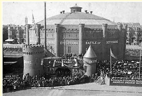
Boston Cyclorama Building
