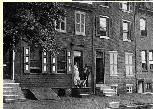
The Whitman House 328 Mickle Street Camden
