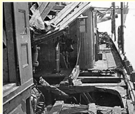
Damage to the CSS Teaser
