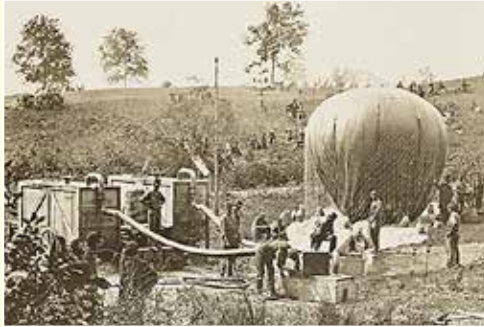
Hydrogen generators filling the Intrepid
