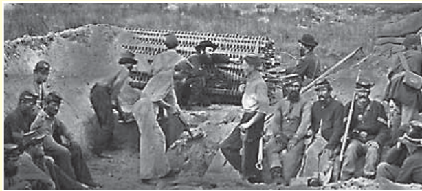
A Union sapper or combat engineer group digs a trench in the direction of an enemy fortification. A gabion provides cover from enemy fire. At Port Hudson a sugar hogshhead stuffed with cotton or a cotton bale would serve the same purpose.
