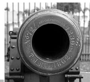
12 Pound Napoleon Cannon of the 1st United States Artillery, Battery H The tube (barrel) has a dent from a Confederate shell. The dent is on the bottom side because the tube was remounted upside down. The gun was made by the Revere Copper Company
