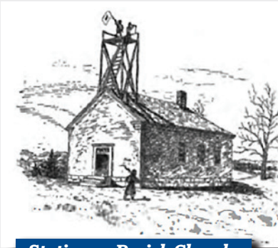
Station on Parish Church, Yorktown
